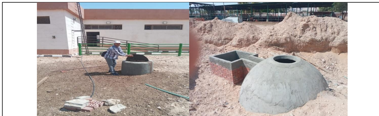
1- Building biogas generating units from organic waste (Sohag University)
