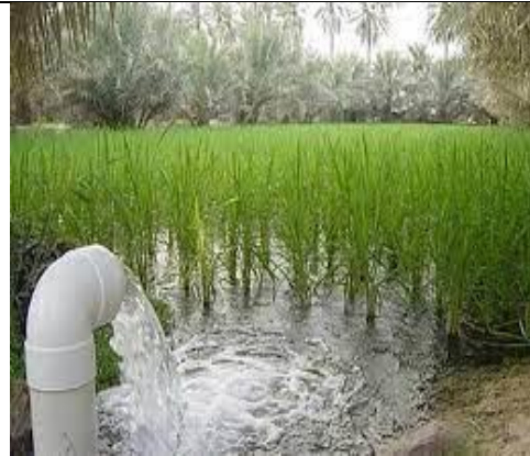
The well After being built
