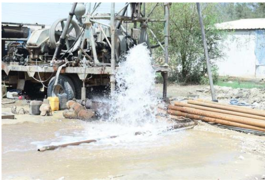
The well after being dug
