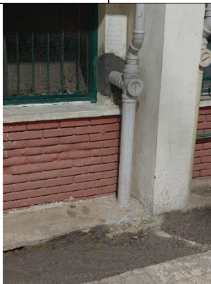
maintenance work for bathrooms
