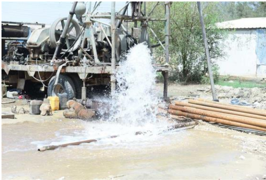
The well after being dug
