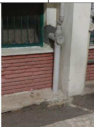
maintenance work for bathrooms
