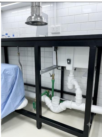
Suspended drainage at student's laboratories
